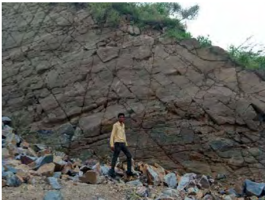
Figure 3.4: Multiple joint sets observed throughout the area.
